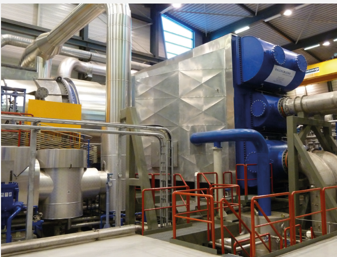
Condenser installed at geothermal power plant in Iceland for district heating and cooling water operation
