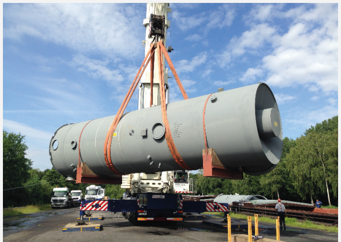
Crane moving MSR at construction site in Finland
