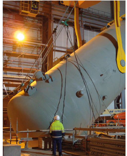
Installation of a new MSR
